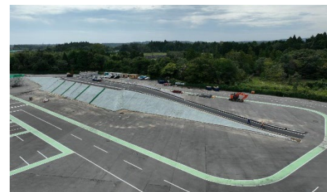
Demonstration test of road fill in the Interim Storage Facility
