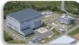
Naraha Center for Remote Control Technology Development
